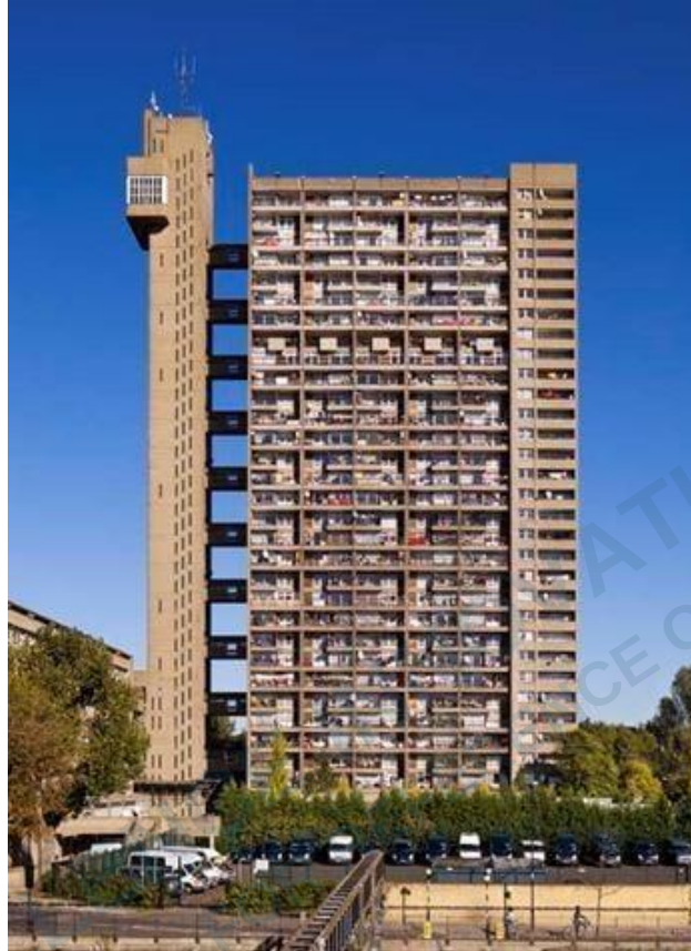
Figure c: Trellick Tower (Source : Historic England Archive)
